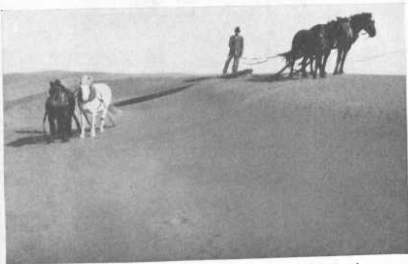
FIGURE 6.—A drag pole being used to break the crest of a dune.
